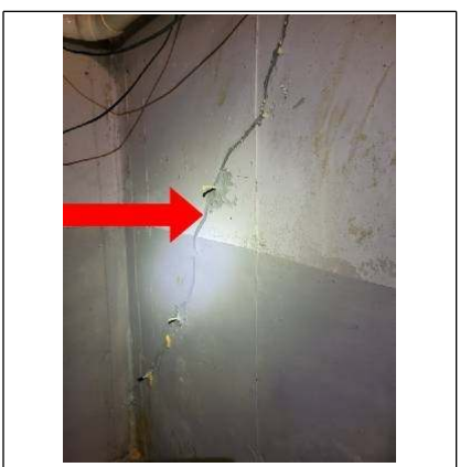
Patch vertical crack in foundation stem wall north side of basement
